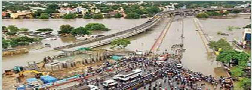
Figure 1- Chennai Floods, 2015 (Source- NITI Aayog)
