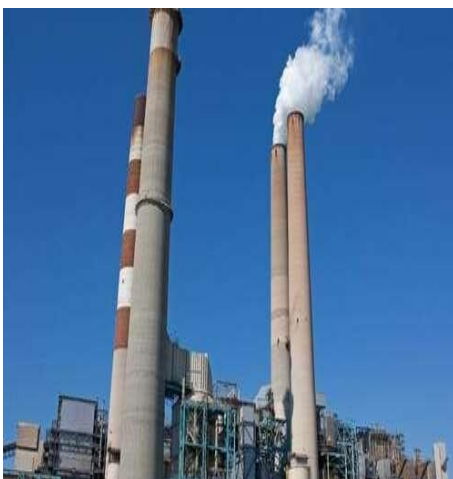
FGD Works at Harduaganj Thermal Power Stations, UP
