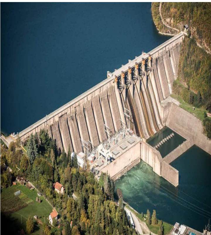
1000 MW Pakal Dul Hydro Electric (H.E) Project on the River Marusudar in District Kishtwar, Jammu & Kashmir
