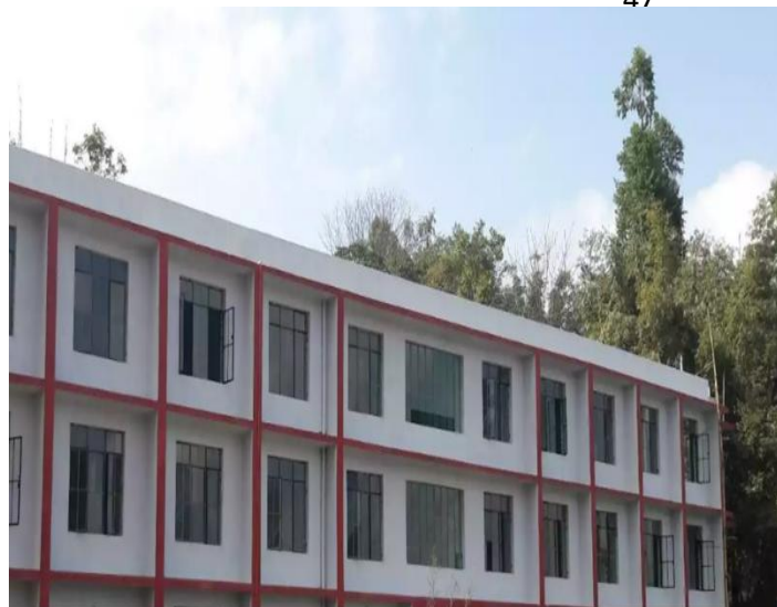
Construction/Infrastructure Development of Kohima College at Nagaland
