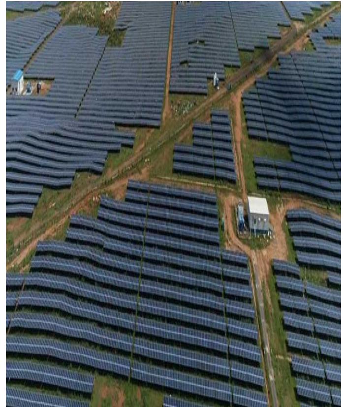
100 MW solar power project at Anantapur Dist., Andhra Pradesh
