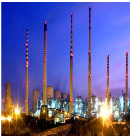
FGD - Bellary Thermal Power Station", Karnataka.
