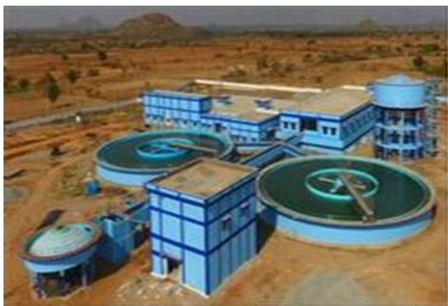
Akbar Nalgonda segment 70 MLD WTP, Telengana
