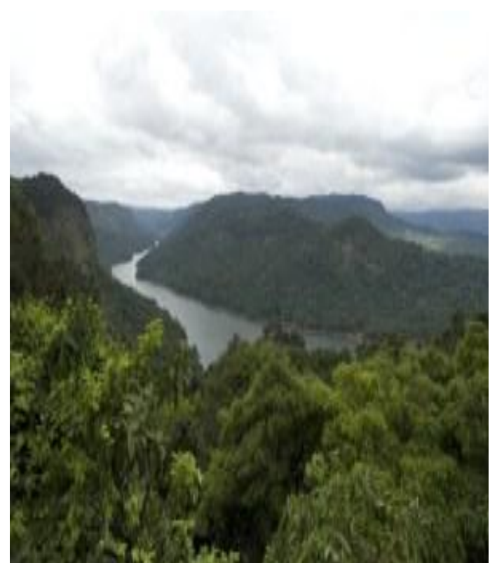
2000 MW Pumped Storage Project at Sharavathy, Karnataka
