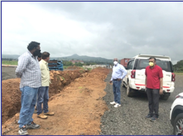
Embankment upto Granular sub bas
