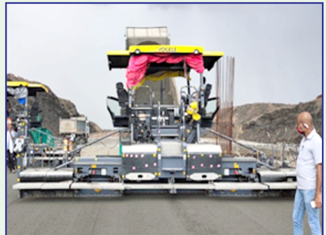
Pavement Quality Concrete laying
