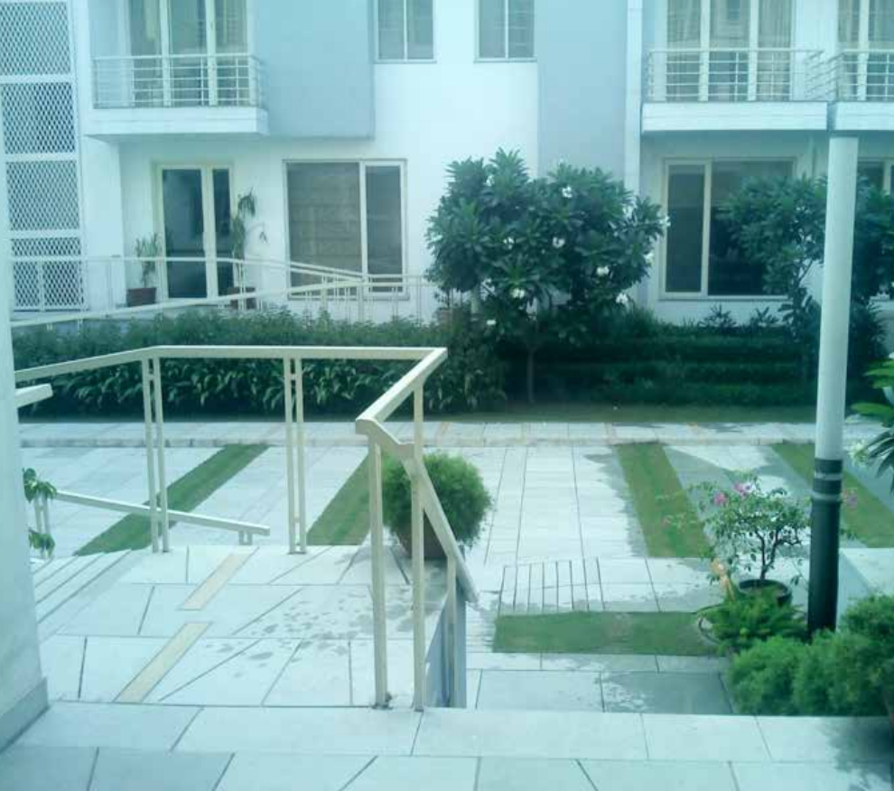
A Combination of Hard and Soft Areas and Ramp with Anti-Skid Flooring
