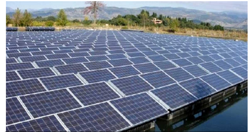
Feeder Solarization Project, Maharashtra
