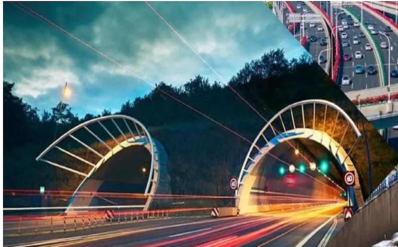
Bengaluru Twin Tunnel Corridor Project
