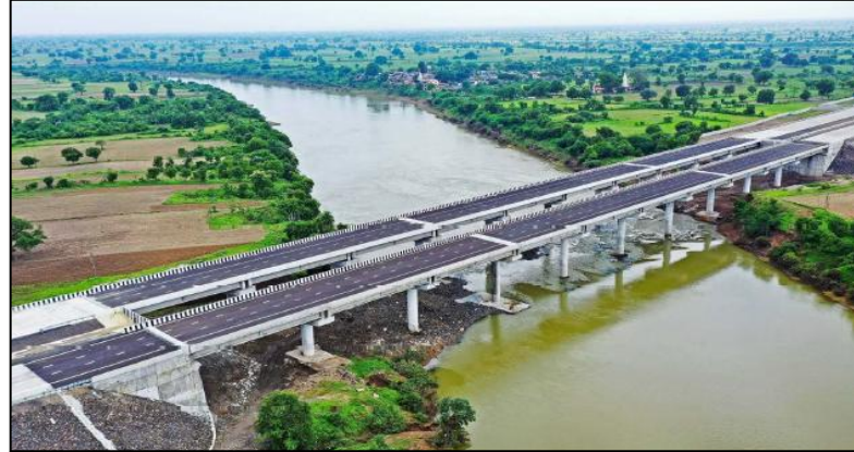
Nagpur Mumbai Expressway, Maharashtra
