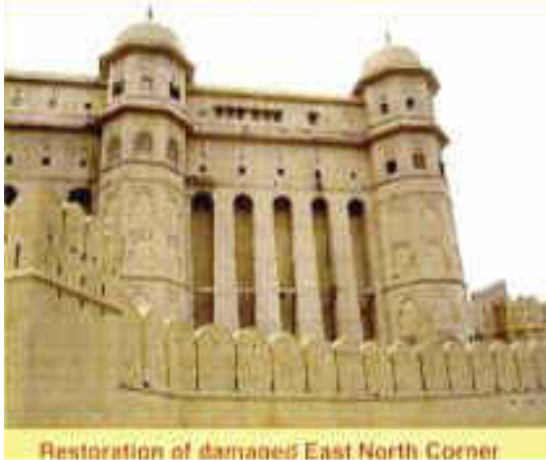
Restoration of damaged East North Corner
