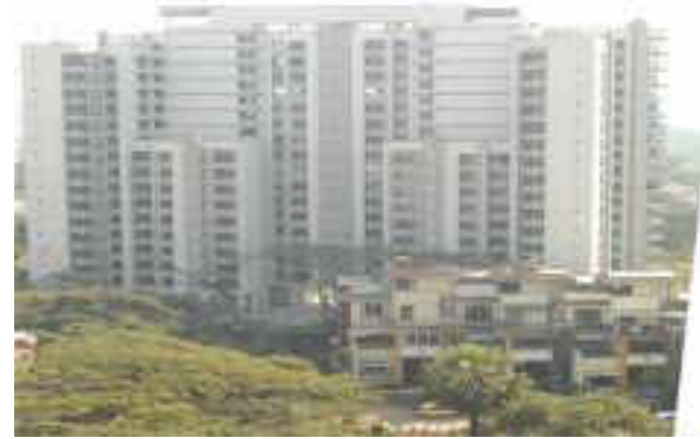
Saptashree Developers, Wagle Estate, Thane incorporates Rain Water Harvesting
