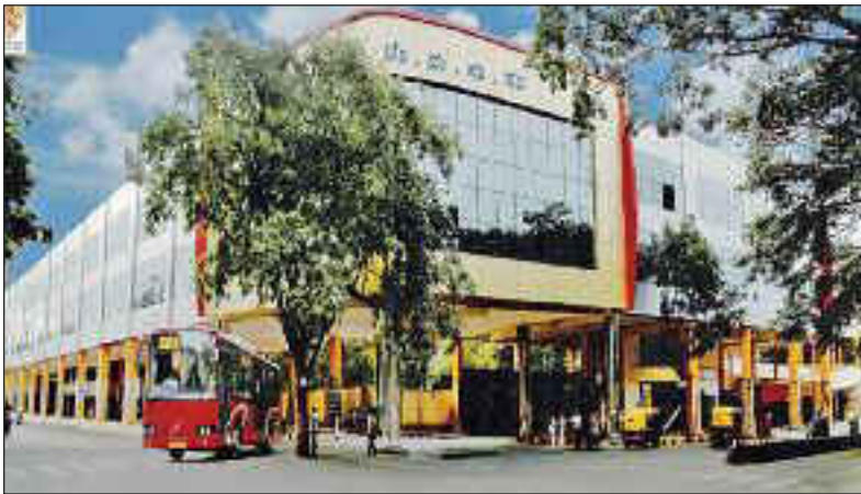
TTMC Jayanagar 4th Block, Project Cost : ₹. 12.90 Crore , Date of Commission:31.8.2009.
