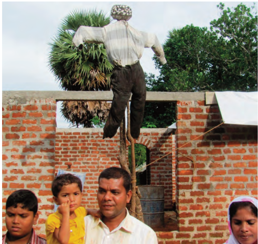
Figure 2: The owner family with their house under construction
