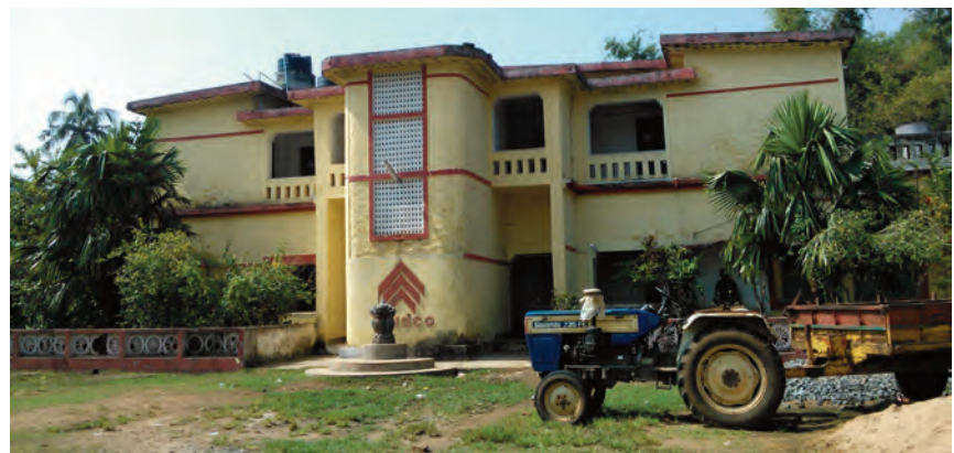
Figure 8: Structure at present
