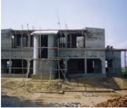
Figure 3: Shelter under Construction
