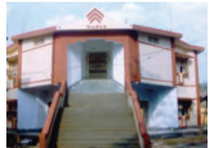
Figure 11: Structure after construction
