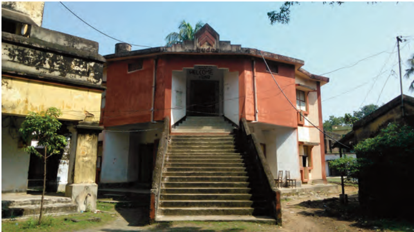
Figure 10: Structure at present
