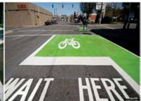
Figure 3: Advanced stop line (7)
